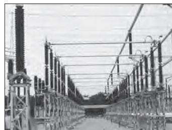
Gelang Patah Substation Project
